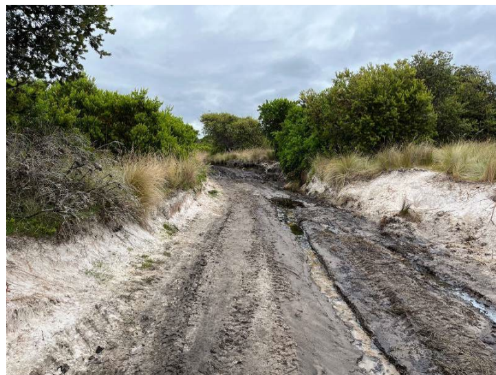
Fig. 55 Restricted road access to Templestowe Beach, being used as public access by a range of vehicles, eroding, drainage impaired and habitat compromised with water quality and sedimentation
